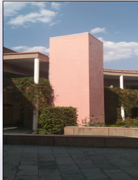
New Lift for first floor
